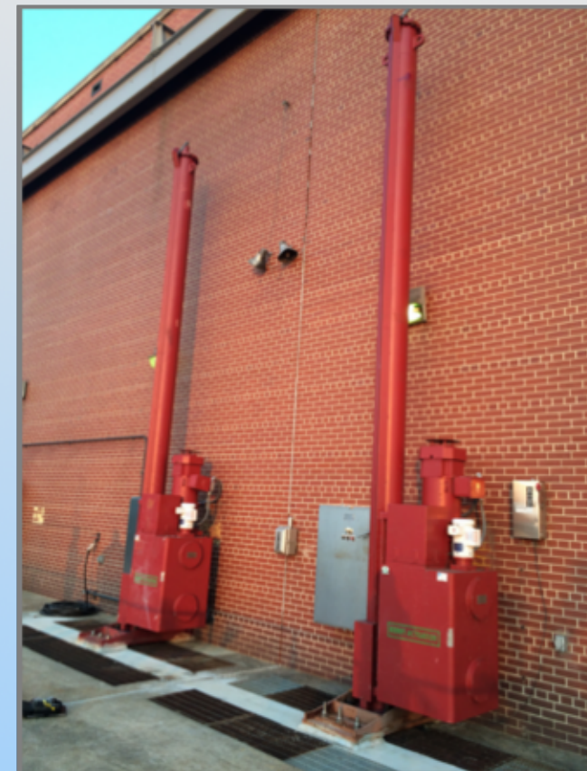
Kerry Actuators on an Isolation Sluice Gate Application
