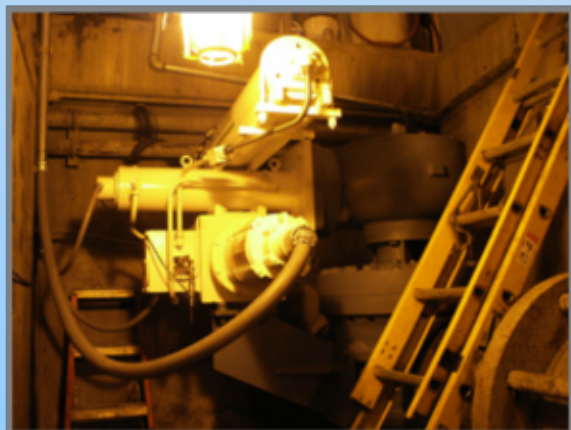
Submersible Kerry Actuator Operating a Cone Valve
