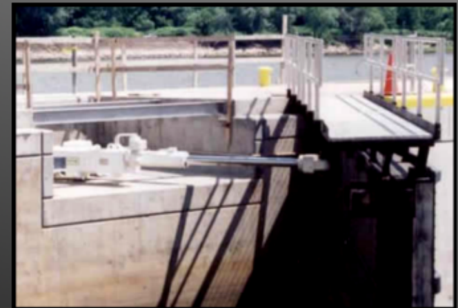
Submersible Kerry Actuator Operating a Lock Mitre Gate
